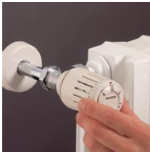
The head is now fitted and the valve can be reopened to the required number setting.
